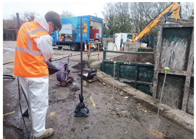
Above: During resin injection
