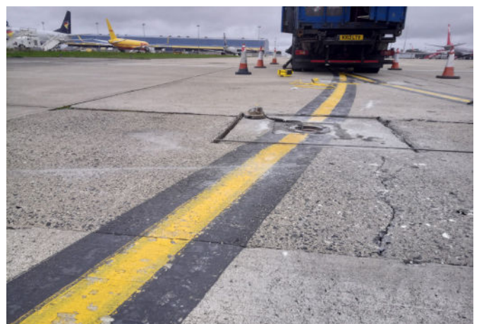
Taxiway "after" resin injection
