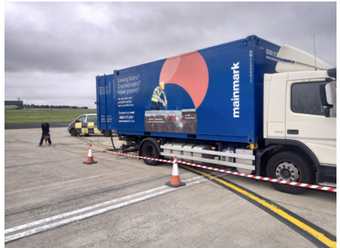
Resin injection being carried out on the taxiway
