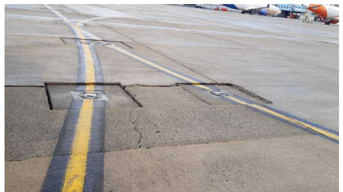
Taxiway "before" resin injection
