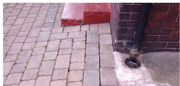
Corner of house re-levelled
