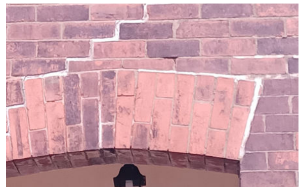
Step crack closed up and repaired
