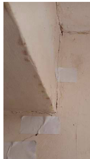
Crack on wall closed after Teretek treatment
