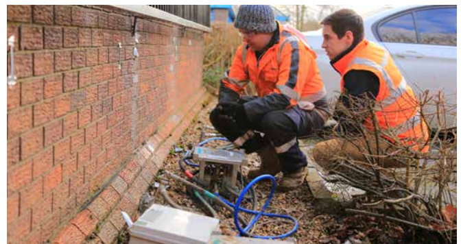
Mainmark engineers monitoring non-invasive re-levelling
