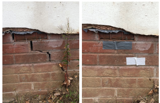
Wall crack before and after Teretek® engineered resin being injected
