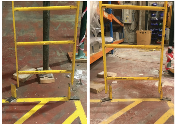
Ladder positioning before and after re-levelling work with Teretek® resin injection
