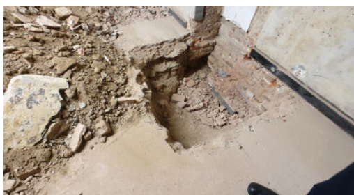
Trial pits exposing existing foundations and ground conditions of site
