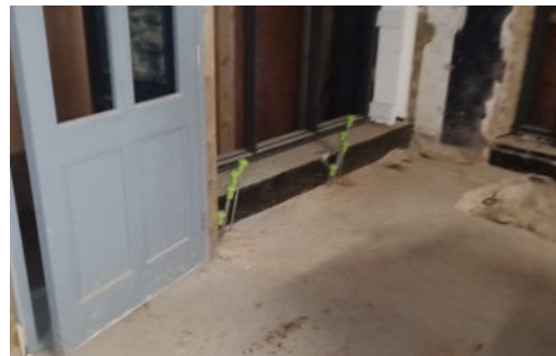
Injection points underneath foundation at front wall
